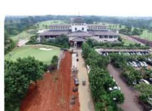
Staging Area Under Renovation
