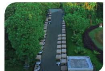
Widening Staging Area
